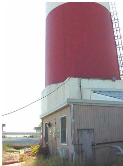
Figure 3-3. Building 715 – Stack Monitoring Facility
