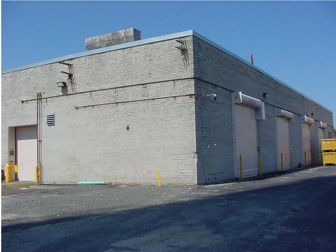
Figure 3-1. Building 704 Fan House
