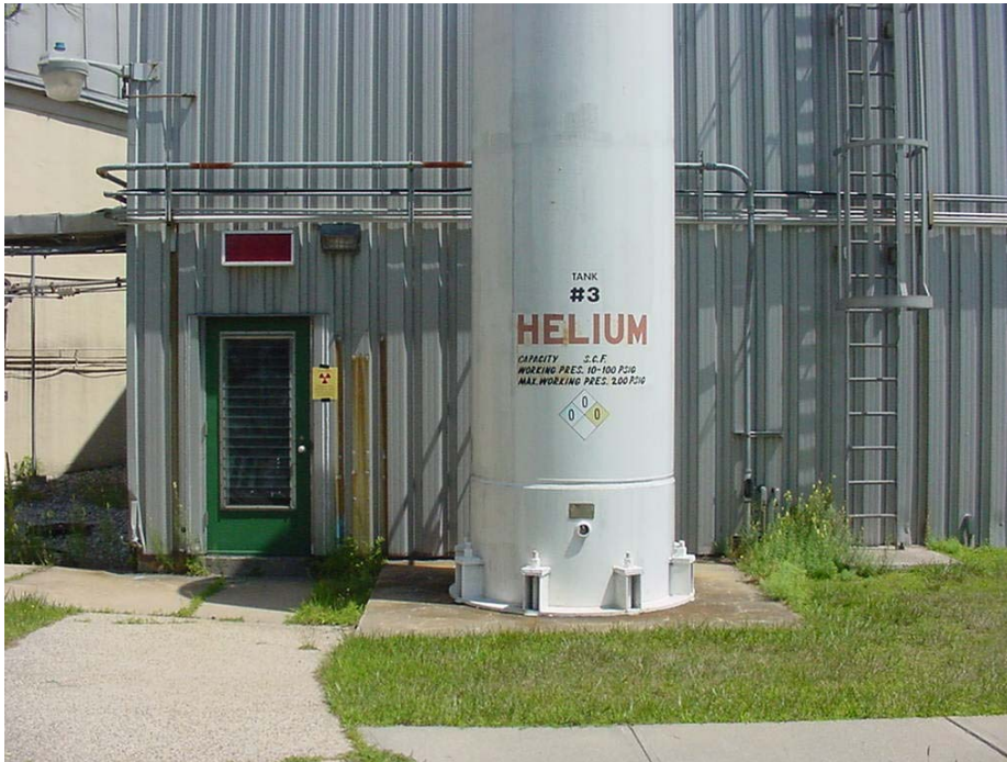
Figure 3-4. Building 751 – Cold Neutron Facility
