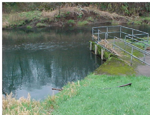
Seasonal use of surface water sources can significantly affect DBP levels.
