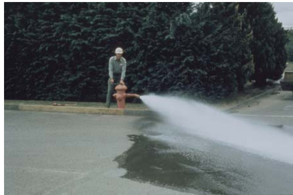
Flushing the distribution system.
