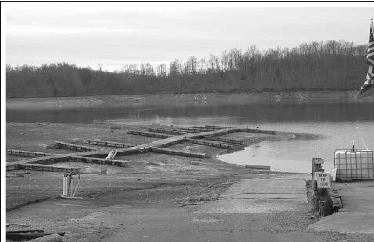
Boat docks sitting on exposed reservoir bottom at a marina on Boone Reservoir
