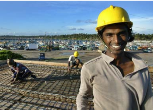
Sri Lankan construction workers helping to rebuild the Dondra Harbor
