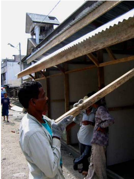
Banda Aceh Market Rehabilitation laborer at work. Photo: Paul Dillon from International Organization of Migration/Banda Aceh
