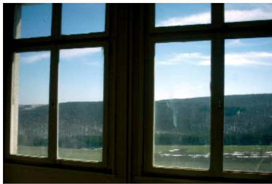
Window weatherstripping at Omurtag Hospital in Bulgaria.
