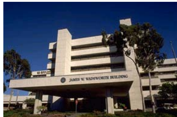
VA Medical Center West Los Angeles, CA, 1976 (not VAHBS, used interstitial space)
