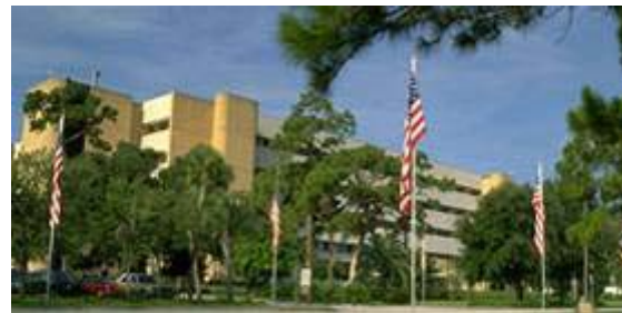
VA Medical Center Bay Pines, FL, 1983
