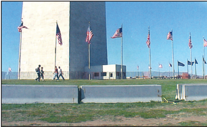
Figure 5: Modifications to Physical Security Enhancements of the Washington Monument
