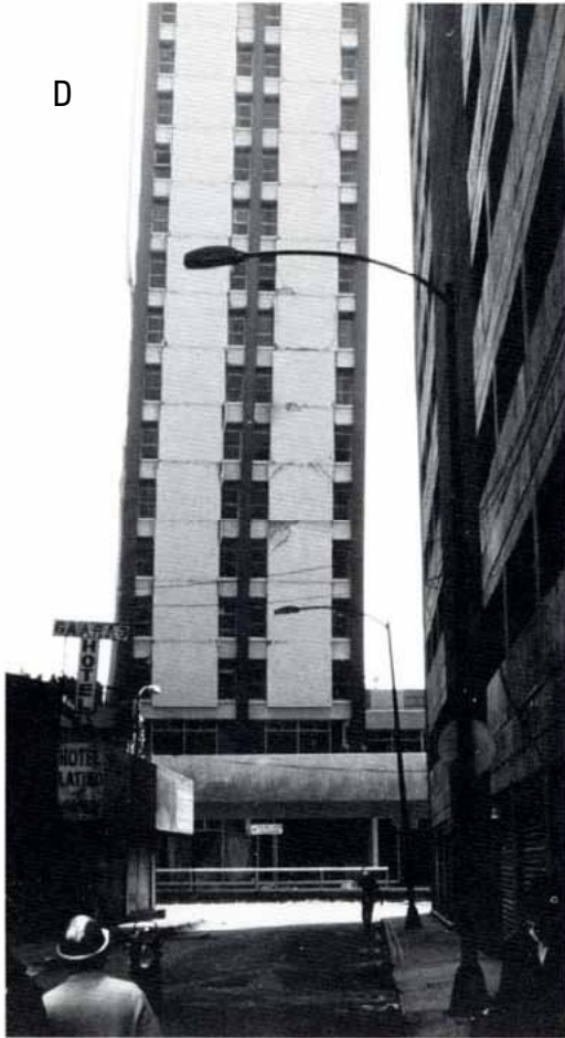
Figure 4-7. Damage in Mexico City, September 19, 1985, from an earthquake some 200 km distant. (A) Collapse of a 21-story building on top of a 14-story building in the Pino Suarez complex. Three towers are left standing with extensive damage to the two 21-story towers. Source: Bob Reitherman; (B) Failure in the welds connecting the flanges and webs of built-up box column possibly led to local flange-buckling of the column and eventual collapse. Source: Bob Reitherman. (C) Debris of tower collapse spilled on to the streets. Source: Mehmet Celebi, USGS. (D) This 21-story steel building remained standing, but was leaning six feet out of plumb at the roof level due to yielding that resulted in a permanent interstory drift (Source: Jim Beck, Caltech). Such permanent tilting would most likely render the vertical transportation system (elevators) unusable due to misalignment. In addition, doors to staircase shafts may be jammed due to deformation of the frames, possibly hampering evacuation efforts.
