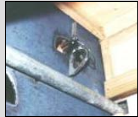
Anchor Point Assembly in training mock-up
