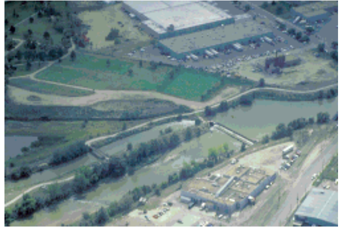
The Burlington Canal can remove all the flow from the South Platte River near Denver, Colo.
