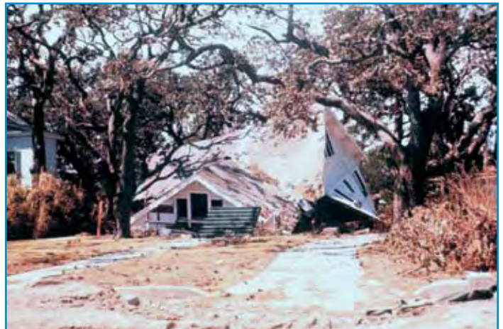
Damage from Hurricane Camille, August 17, 1969/NOAA
