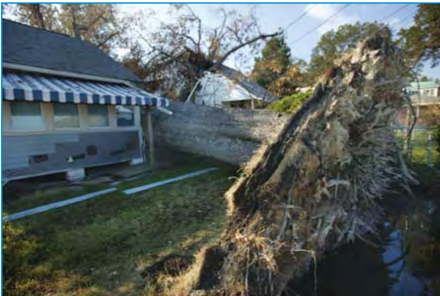
Hurricane Isabel wind damage, Colonial Beach, VA September 30, 2003/ Photo by Andrea Booher/FEMA
