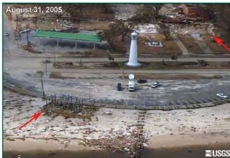
After Hurricane Katrina August 31, 2005— Biloxi, MS/USGS
