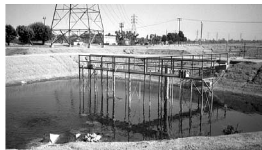
Research basin and catwalk
