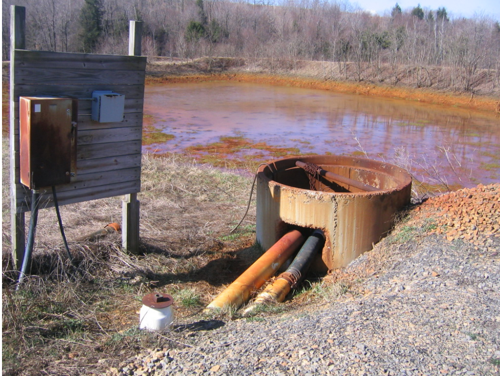
Figure 7-4. Photograph of the Chimney Sump and Collection Basin at PBS Coals Job #8 Source: Site Visit Report Pennsylvania Coal Mine Acid Drainage Treatment Systems (ERG, 2006)
