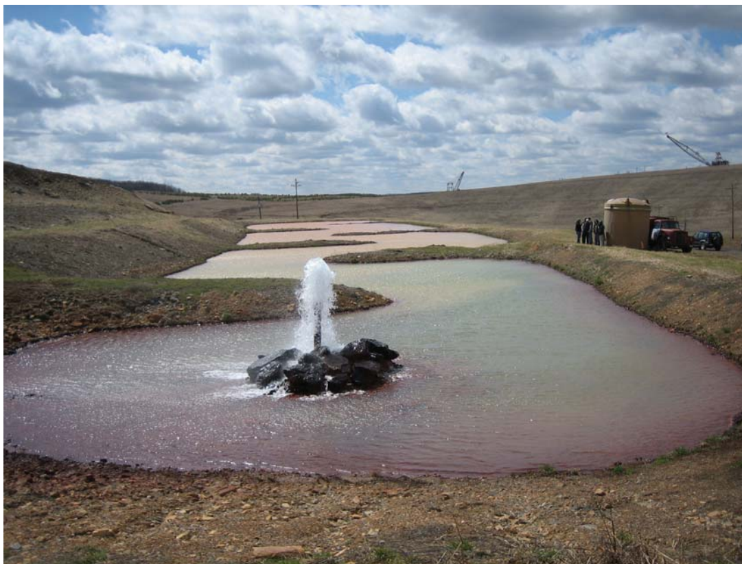
Figure 7-1. Photograph of the Outfall 003 Treatment System Aeration Pond
