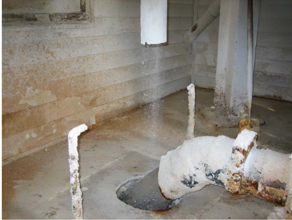
Figure 7-3. Photograph Inside the PBS Job #1 Lime House: AMD Flow and Lime Addition Source: Site Visit Report Pennsylvania Coal Mine Acid Drainage Treatment Systems (ERG, 2006)
