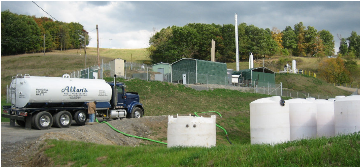
Truck Collecting CBM Produced Water From Tank Battery (Greene County, PA)
