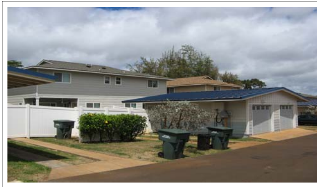
New military housing developed by Actus Lend Lease LLC, including here at Schofield Barracks, feature garages topped with photovoltaic film to generate electricity. The homes also use solar water heaters.
