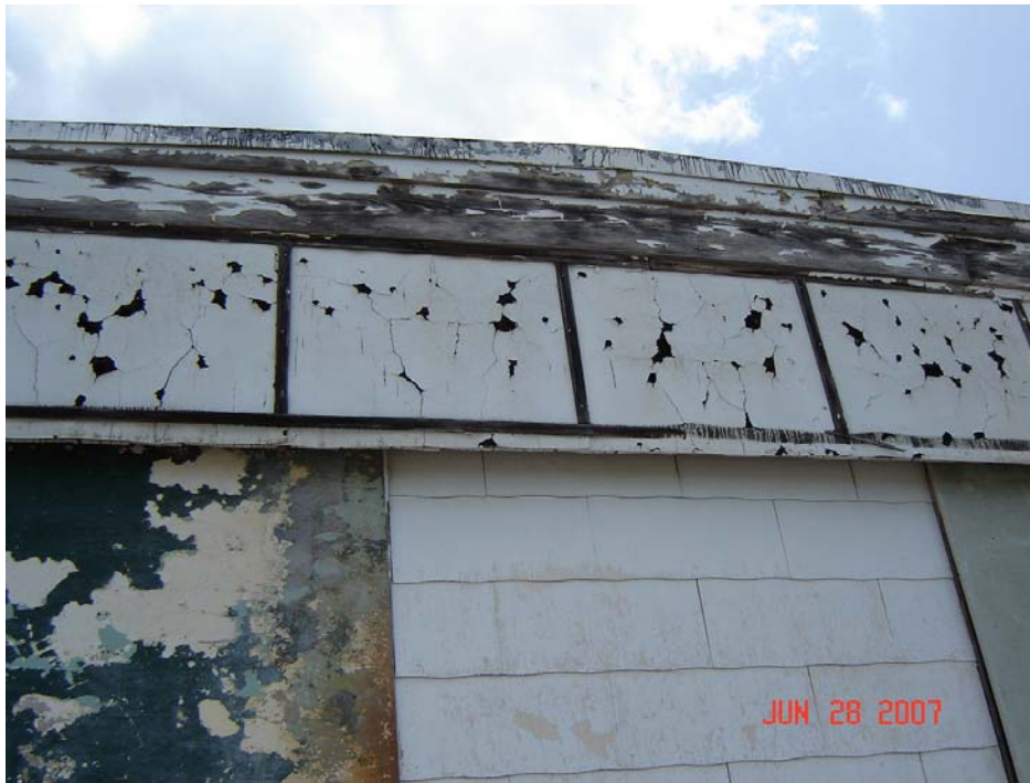
Asphalt Siding on Fascia
