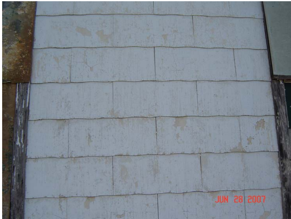
Exterior Transite Siding
