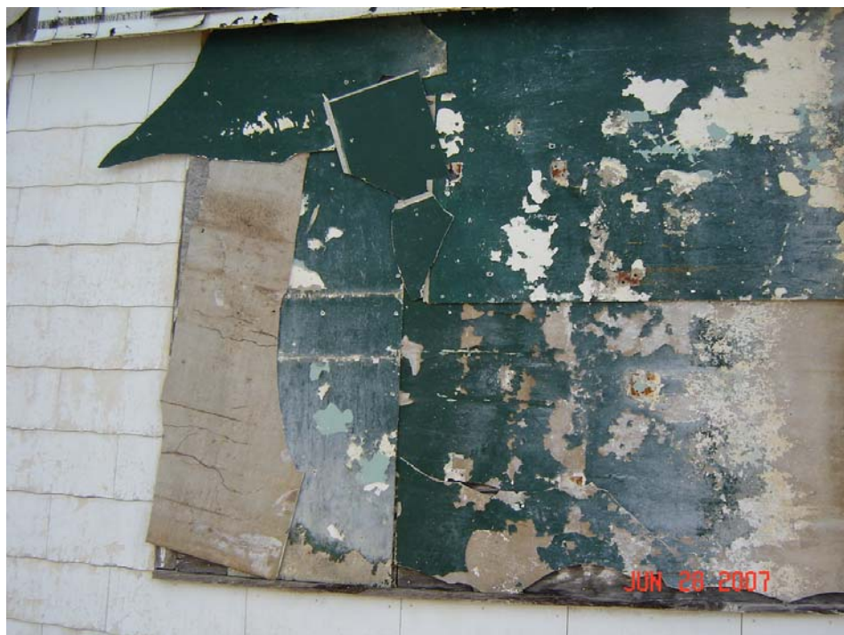
Exterior Transite over Windows
