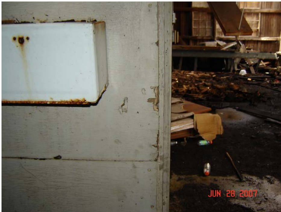
Drywall in Bathroom
