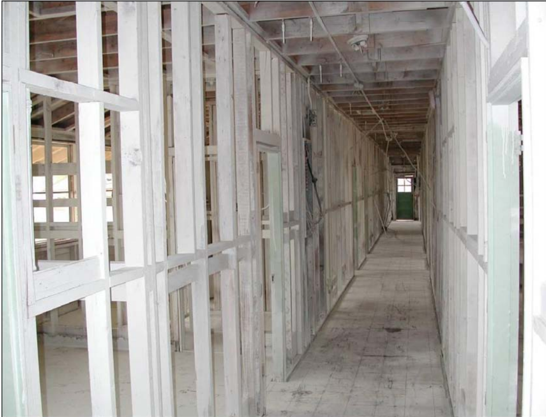
Figure 4-6. Abated area after application of encapsulant.
