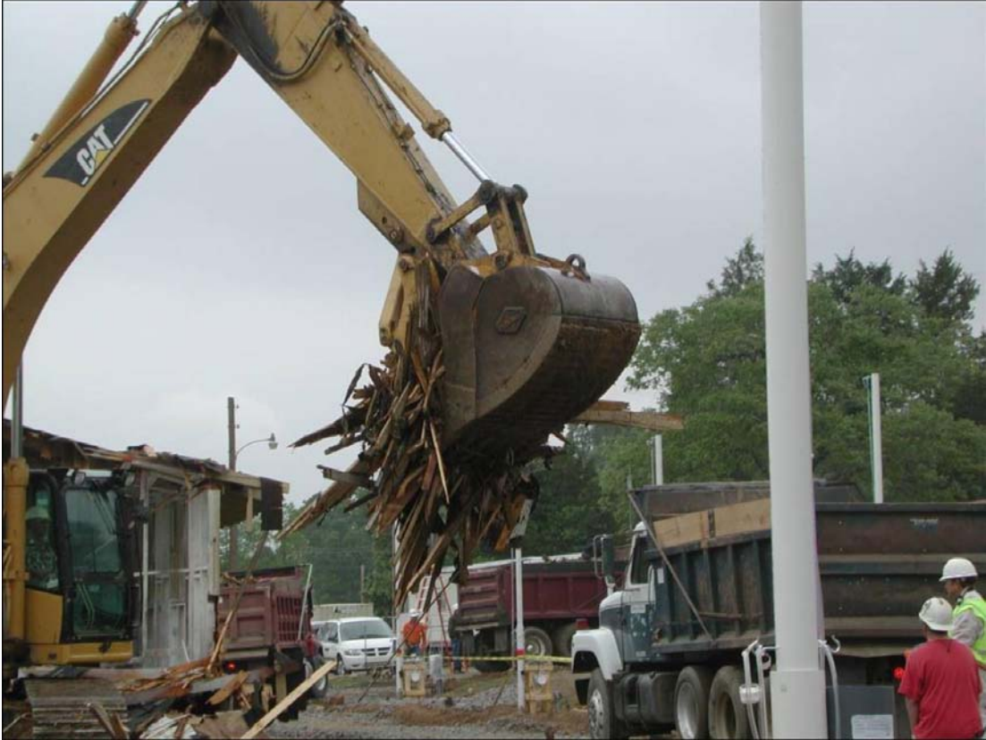
Figure 4-18. Loading NESHAP debris into trucks.
