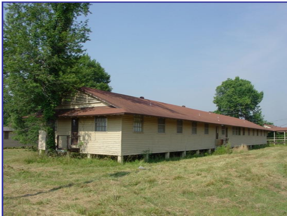
Figure 3-2. (Top) Exterior view of Building #3602 (NESHAP Method) and (Bottom) #3607 (AACM). Dimensions: 30-feet by 150-feet.
