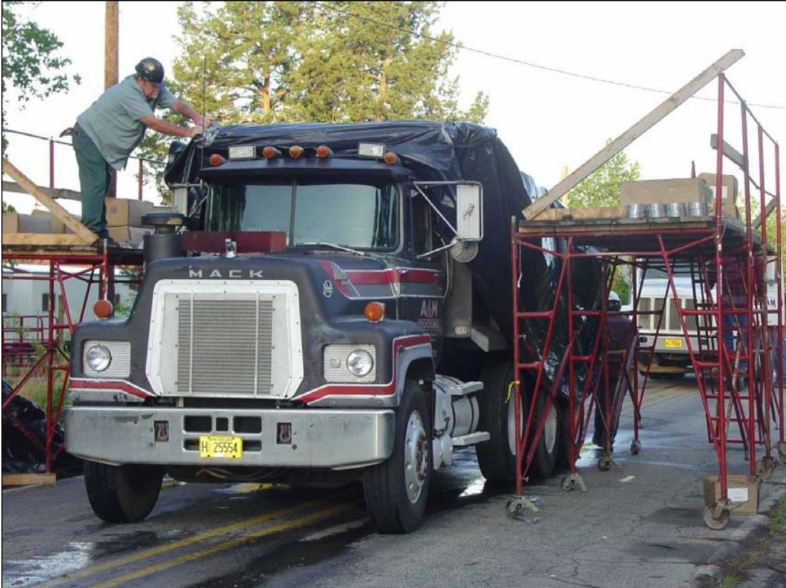
Figure 4-30. Double-lining the trucks for hauling of the AACM debris (View 2).
