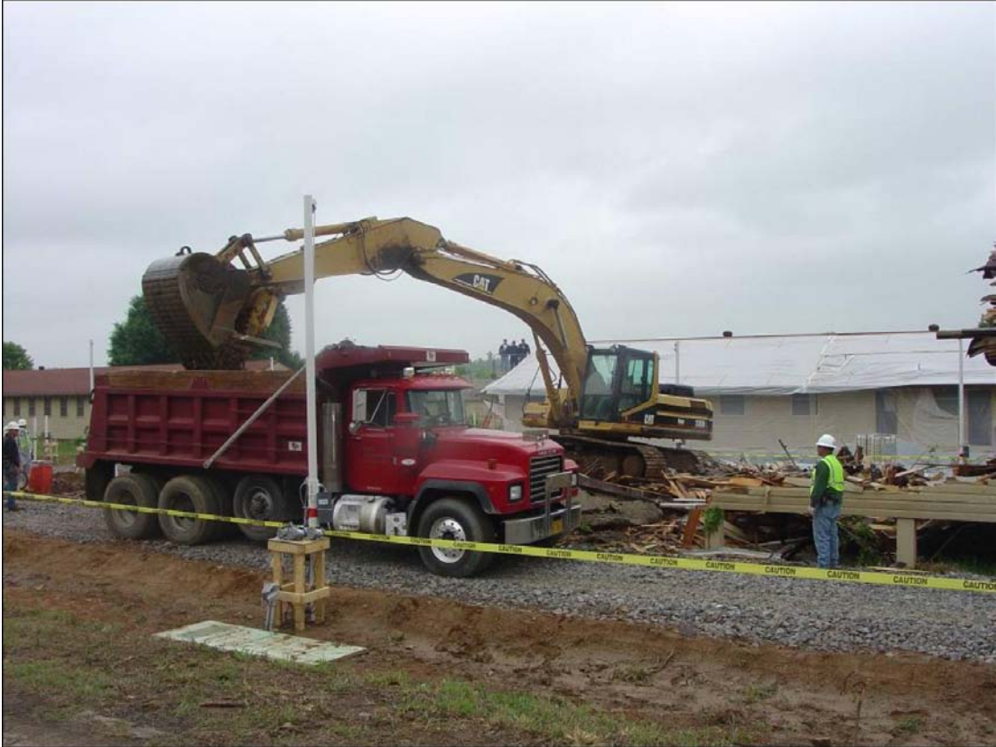
Figure 4-19. Finishing NESHAP demolition.
