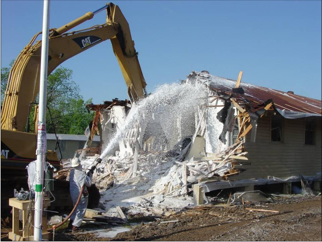
Figure 4-32. Progressing with the AACM demolition.
