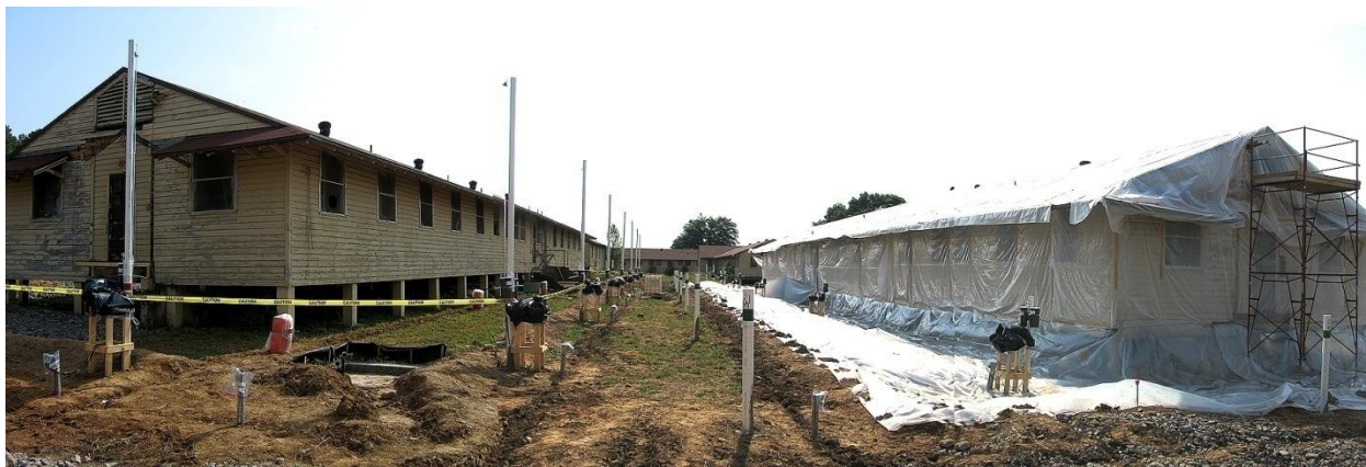
Figure 4-16. Preparation of site prior to demolition of NESHAP Method building (left).
