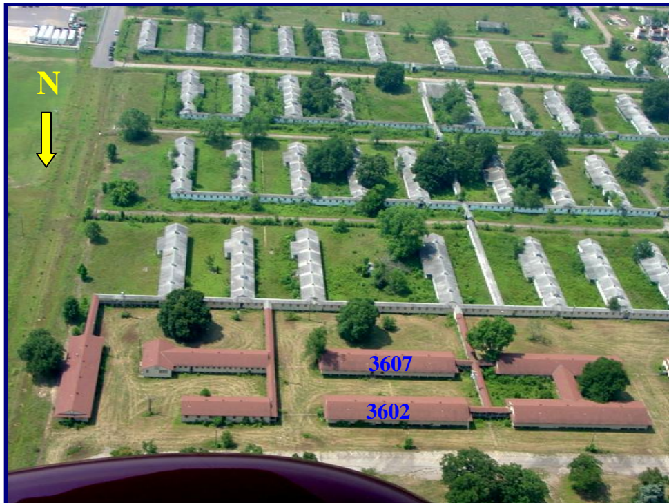
Figure 3-1. Project location at Fort Chaffee. Buildings selected for demolition are #3602 (NESHAP Method) and #3607 (AACM).
