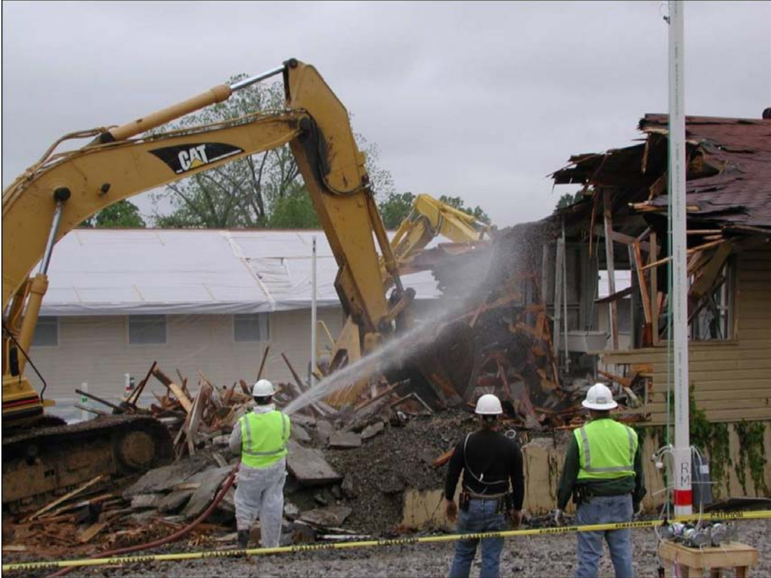
Figure 4-17. Starting demolition of the NESHAP building.
