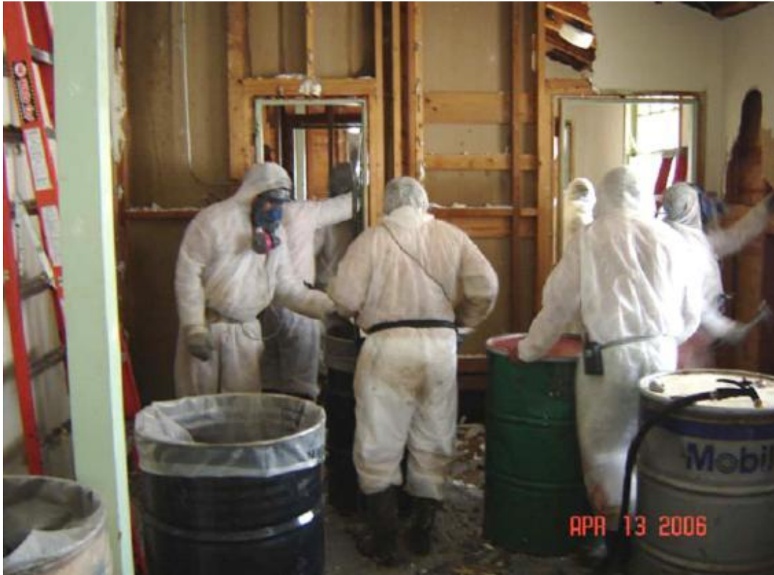
Figure 4-4. Loading abated material into barrels.
