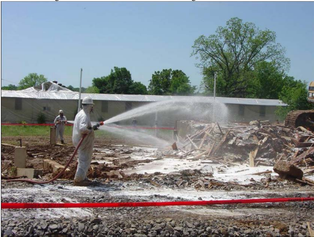
Figure 4-36. Nearing the completion of the AACM demolition.
