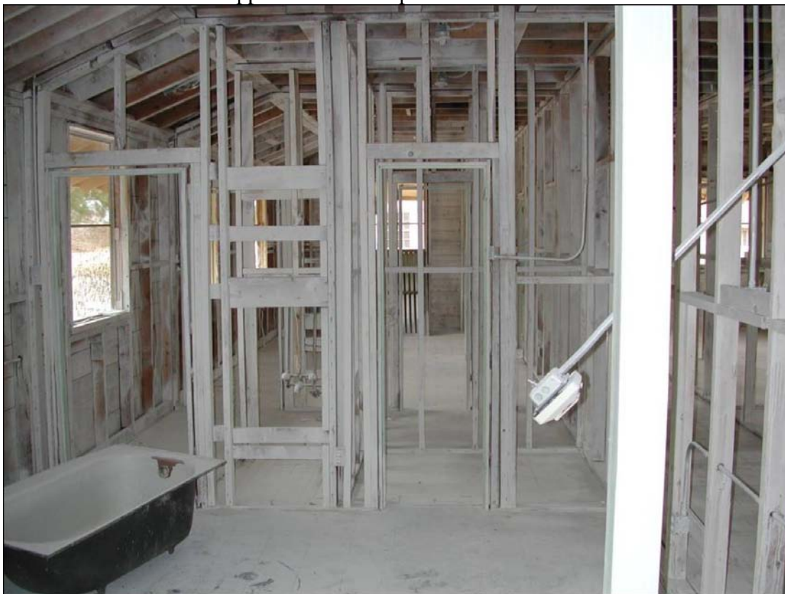
Figure 4-7. Abated area after final clearance.
