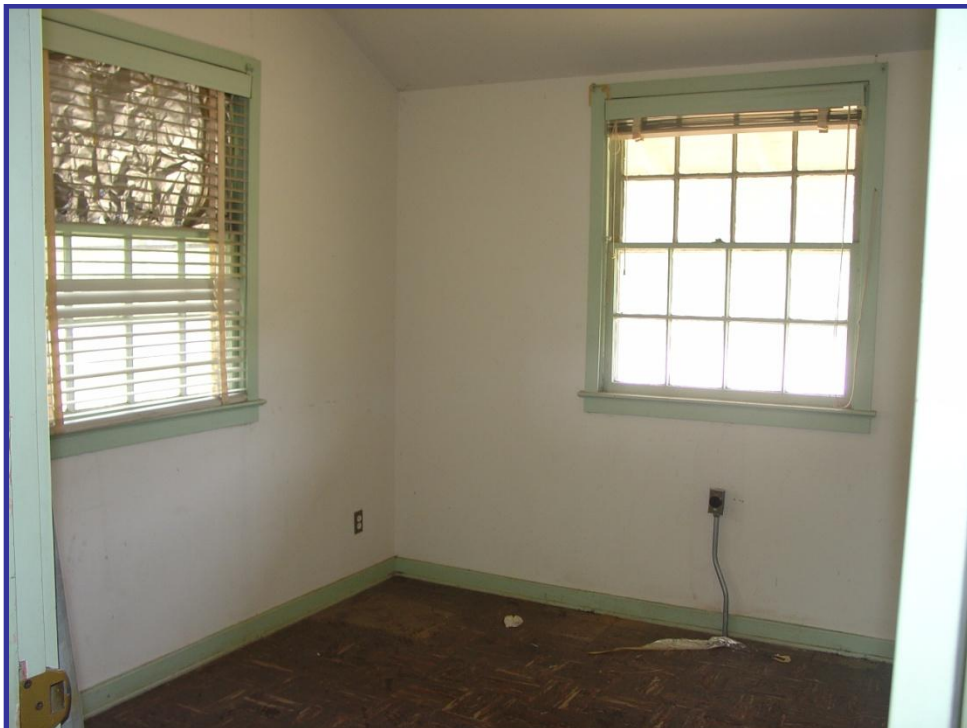
Figure 3-4. Interior view of Building #3607 (AACM). Interior finishes are gypsum wallboard (ceiling and walls) and nine-by-nine-inch resilient floor tile.
