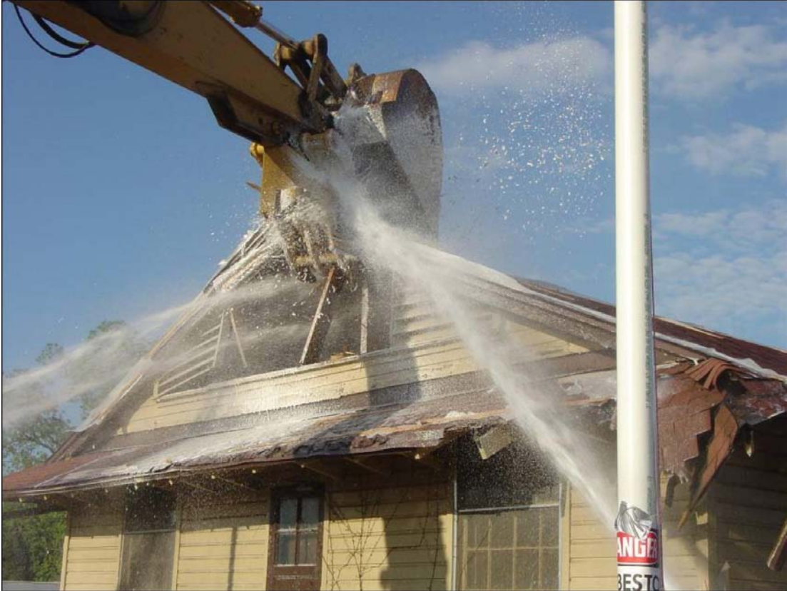
Figure 4-31. Starting the AACM demolition.
