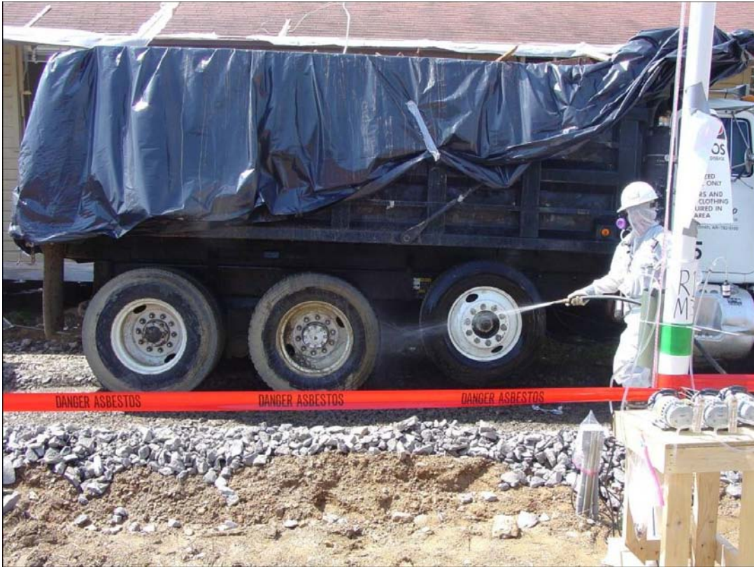
Figure 4-35. Washing the trucks with water before leaving the site.
