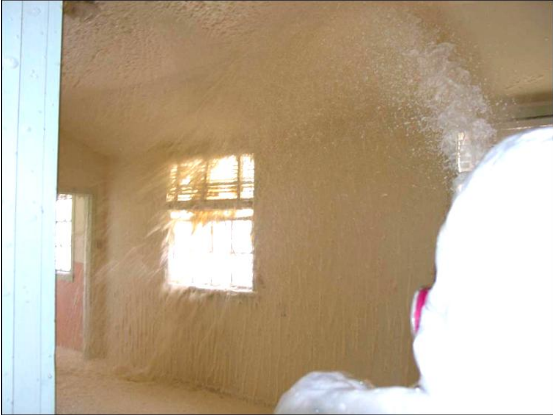
Figure 4-23. Pre-wetting with Amended Water.
