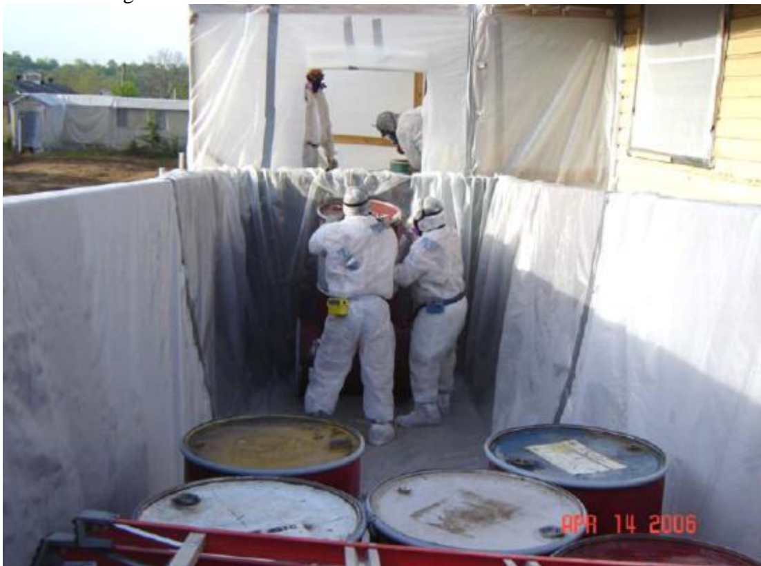
Figure 4-5. Loading asbestos-containing material into roll-off container.
