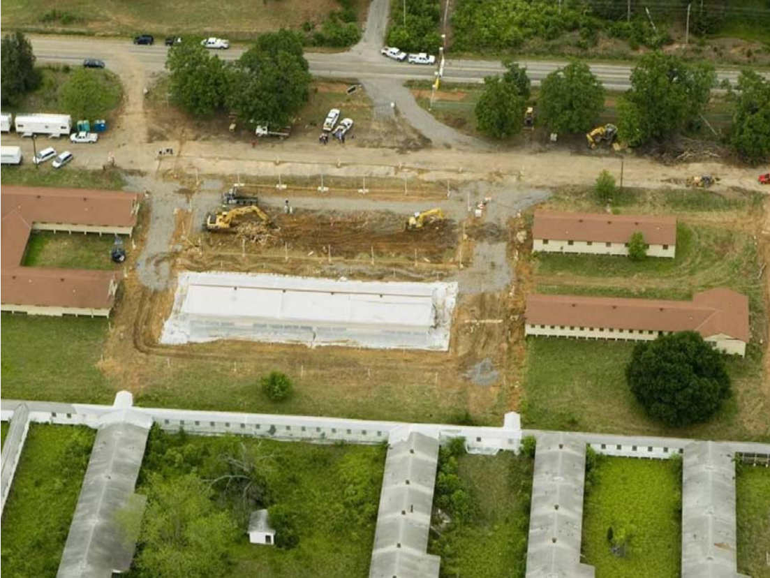
Figure 4-20. Aerial view showing NESHAP building nearly demolished.
