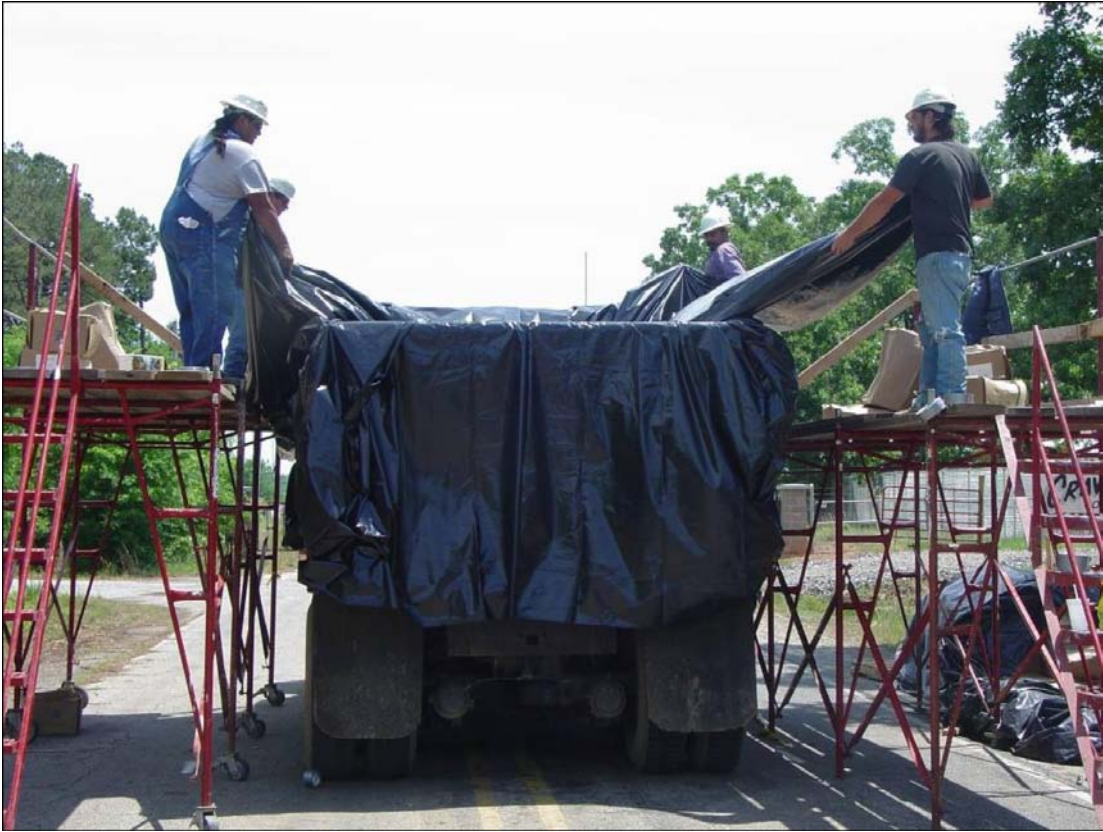
Figure 4-29. Double-lining the trucks for hauling of the AACM debris (View 1).
