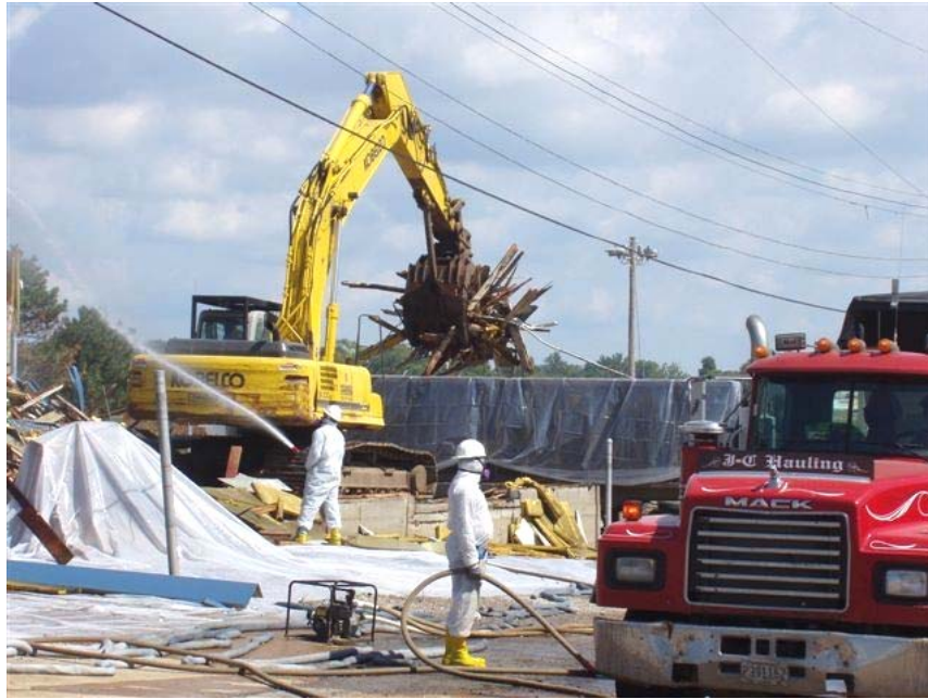
Figure B-2. Transfer of Building Debris to Truck Bed
