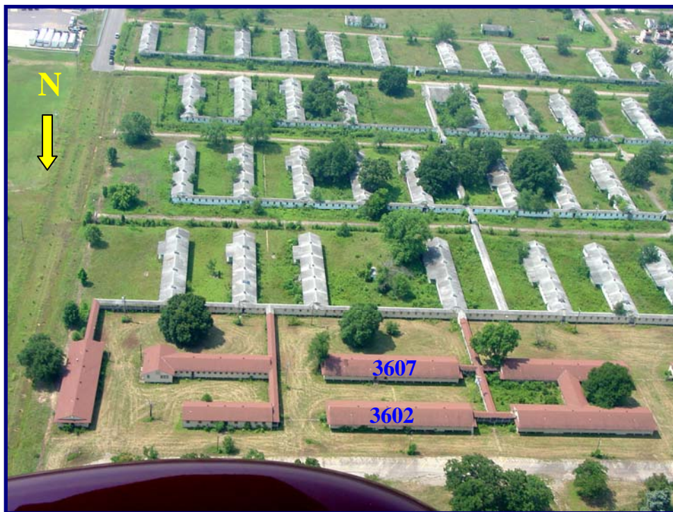
Figure A-2. Aerial view of project location at Fort Chaffee. Buildings selected for demolition are #3602 (NESHAP Method) and #3607 (Alternative Method).
