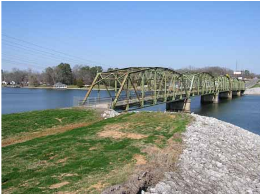
The historic Highway 72 bridge located immediately downstream from proposed site.
