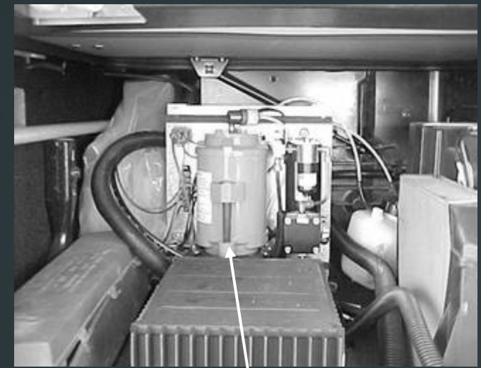
HPCS control reservoir
