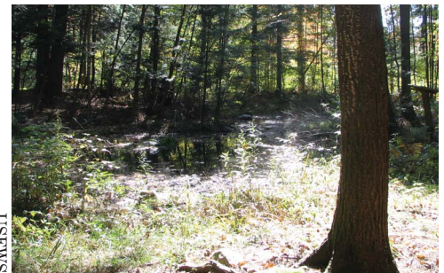
After the cistern's removal, the natural hydrology of this woodland pool is restored and access to wildlife is improved.
