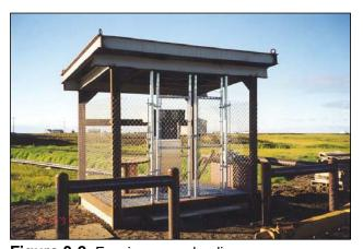
**Figure 3-2**. Fencing around a dispenser pump.
