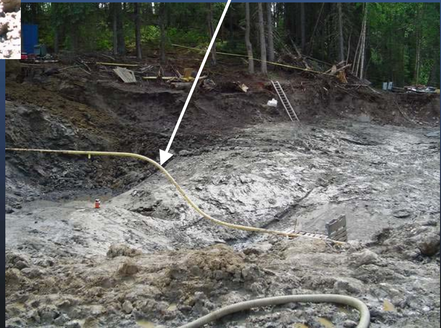
Initial pipeline exposure
