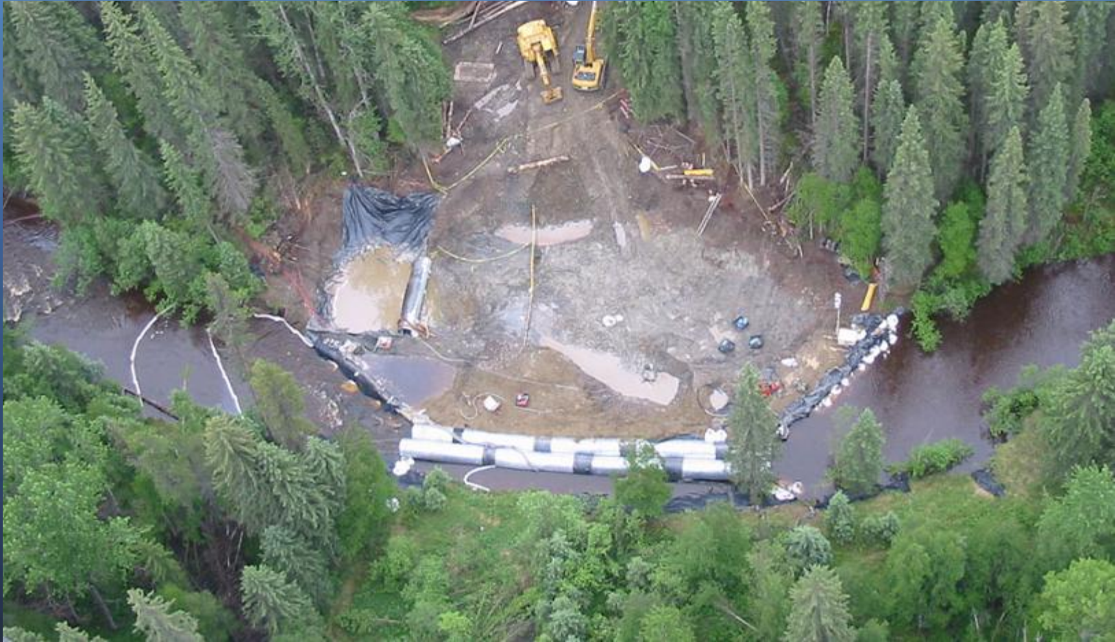
Overview of breakpoint (initial stream diversion in place)
