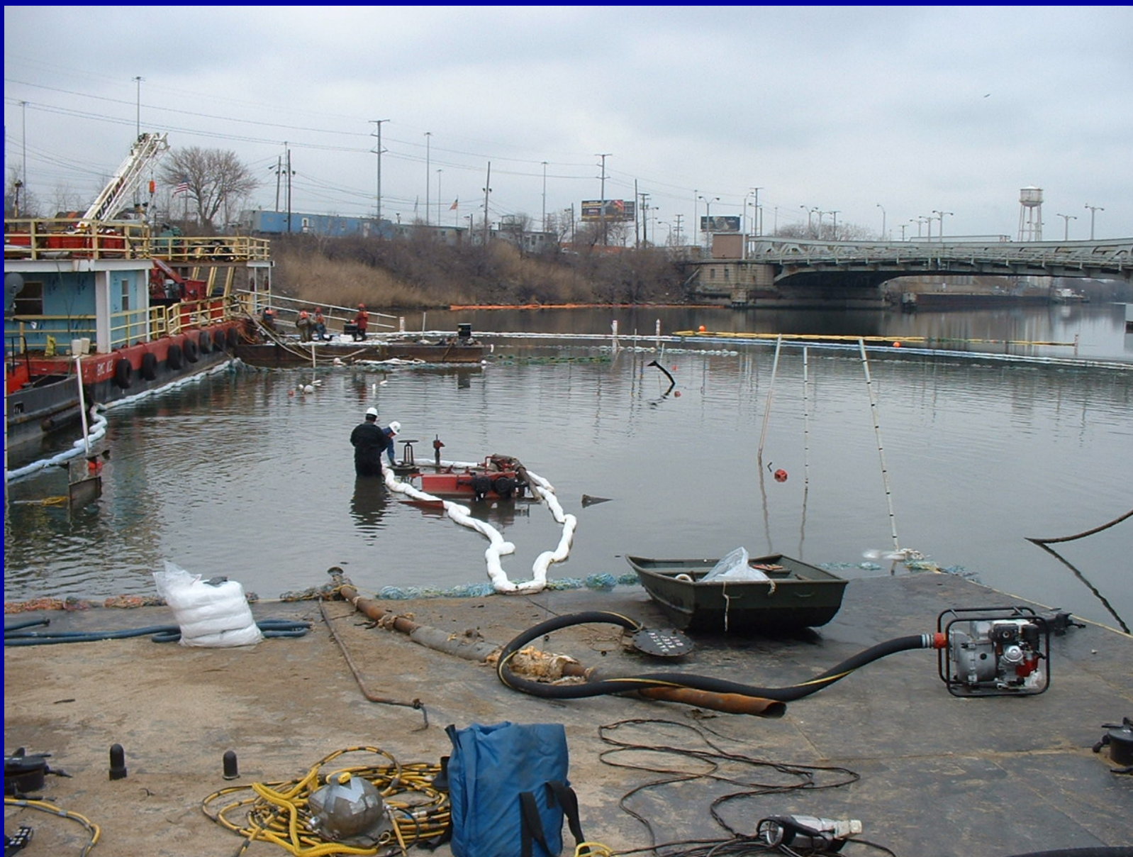
Photo taken from the exposed bow of the barge, with the stern ~295' to the rear and under ~20 feet of water. At this point, all oil is thought to remain on board.
