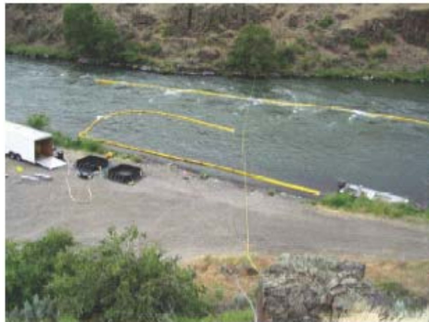
River Mile 42.8a: Looking west from east side road. Note river access and use of trees and rocks to anchor boom.
