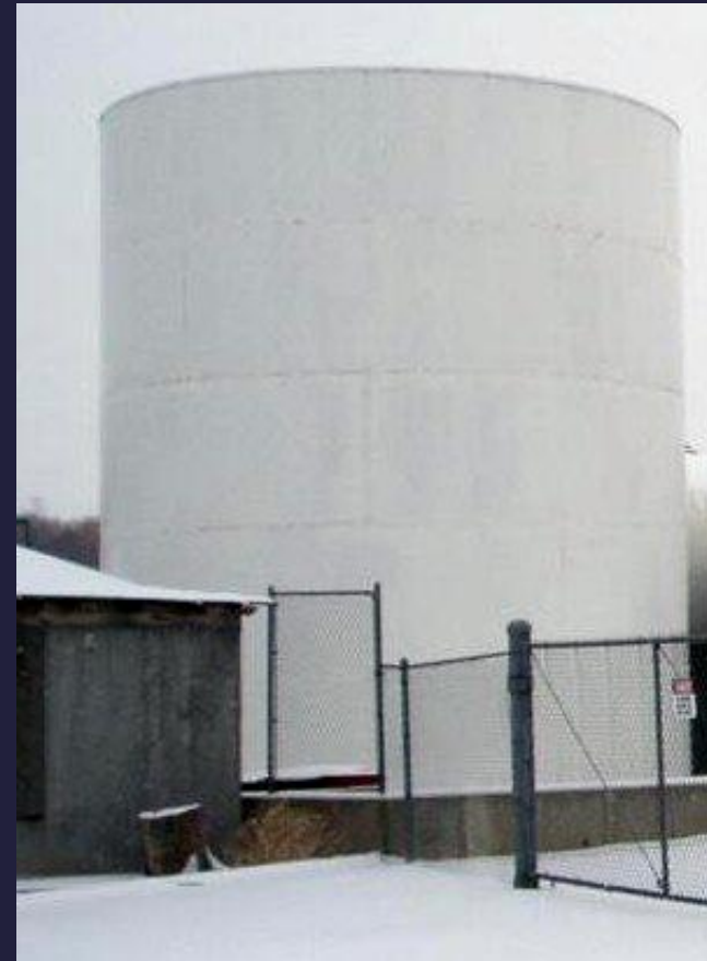
Double-bottom Tank in Concrete Dike
