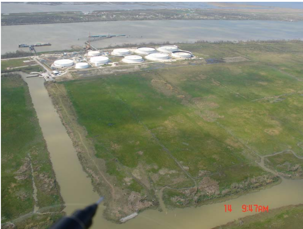
Figure 17. Aerial photo of burn site, March, 16, 2006, 5 months post-burn. Photo credit: Gary Shigenaka (NOAA)
