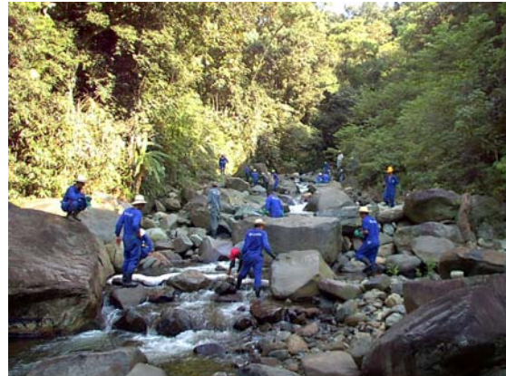
Fig. 22 – Workers in the Rio dos Padres.
