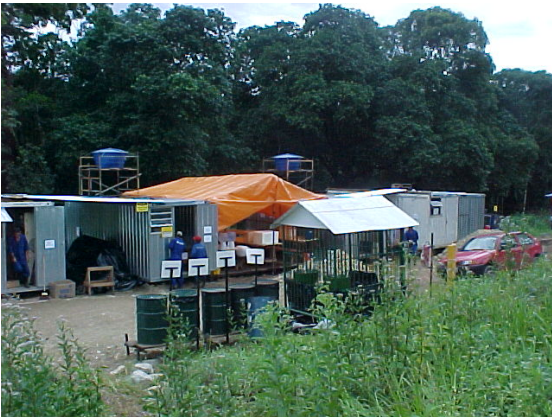
Fig. 15 – Operational base close to the river mouth.
