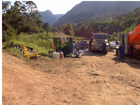
Fig. 16 – Operational base close to the river mouth.
