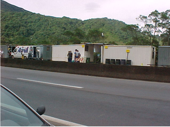
Fig. 13 – Operational base on the roadside.
