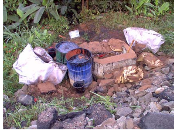
Fig. 8 – Sewer discharge to the forest.
