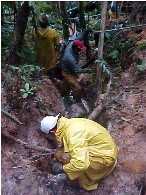
Fig. 17 – Workers cleaning one of the “tracks”.
