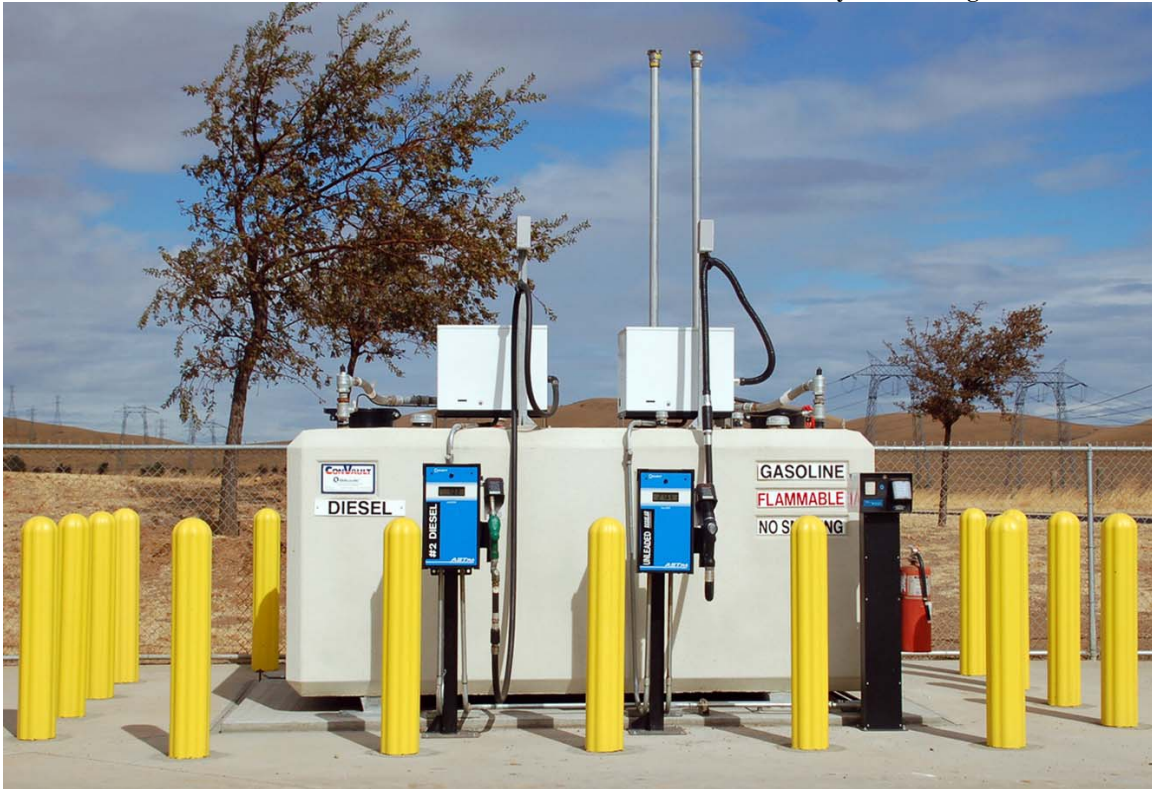
Figure 2 Dual Compartment Convault Protected AST (U.L. 2085)
