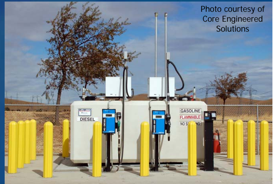
Dual Compartment Convault Protected AST (U.L. 2085)
