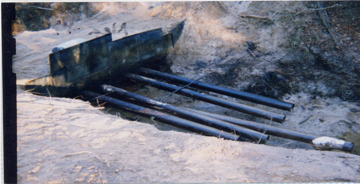
Collins, MS 12/30/99 – 12/31/99 Site: Area 1A Underflow Dam Construction
