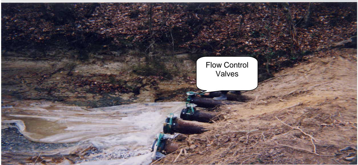
Collins, MS 01/01/00 Site: Area 1A Dam 2 – Underflow Pipes
