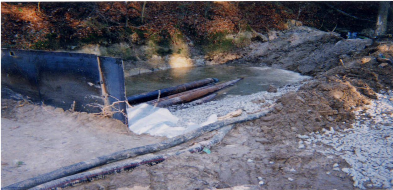
Collins, MS 12/30/99 – 12/31/99 Site: Area 1A Underflow Dam Construction
