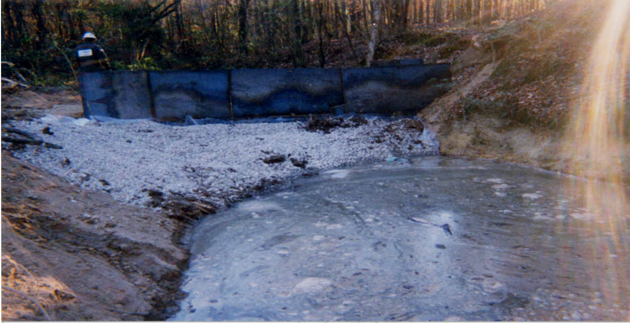
Collins, MS 12/30/99 – 12/31/99 Site: Area 1A Dam Construction
