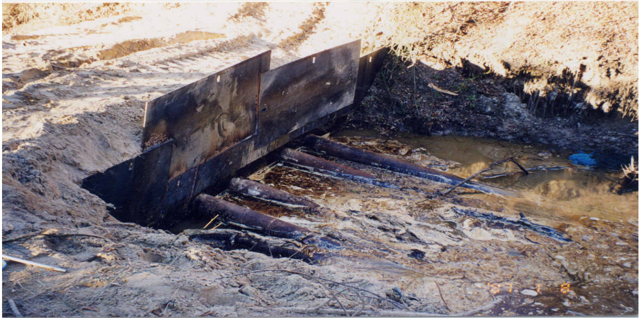
Collins, MS 12/23/99 Site: Area 1A Dam 2 – Underflow Pipes
