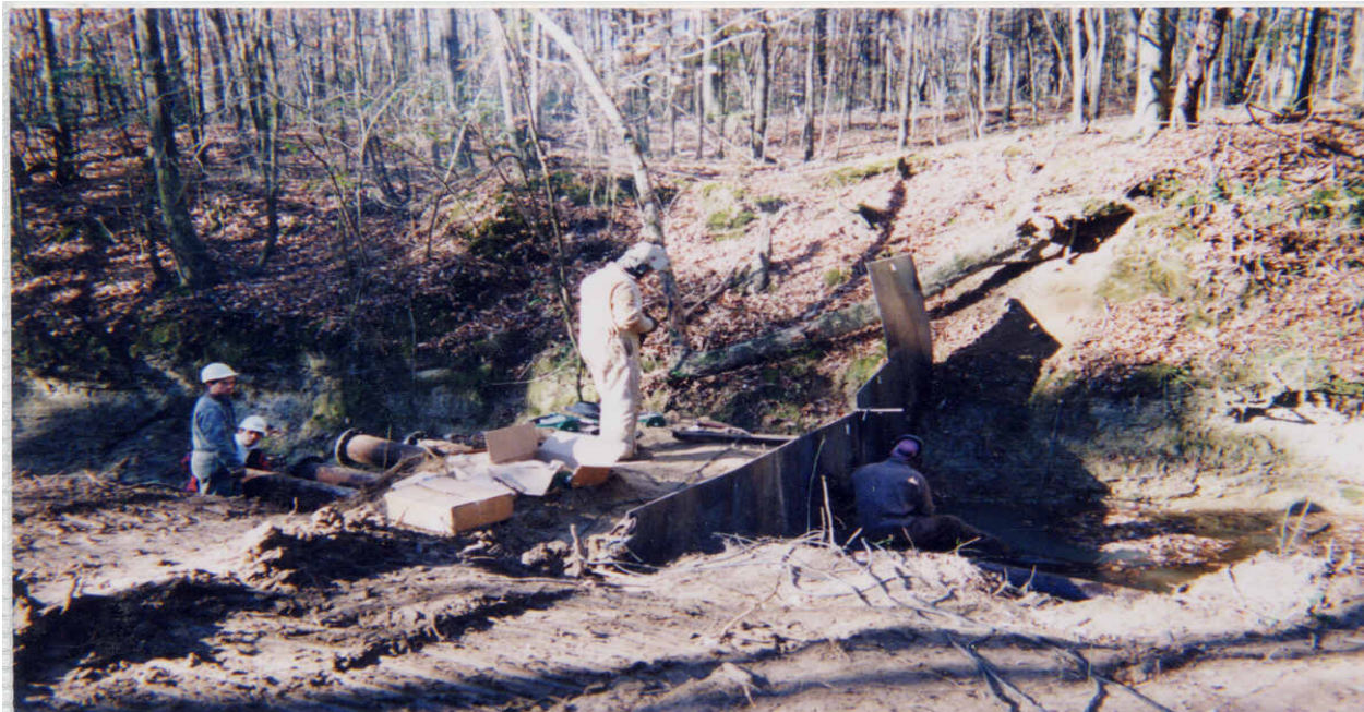
Collins, MS 12/31/99 Site: Area 1A Dam Construction
