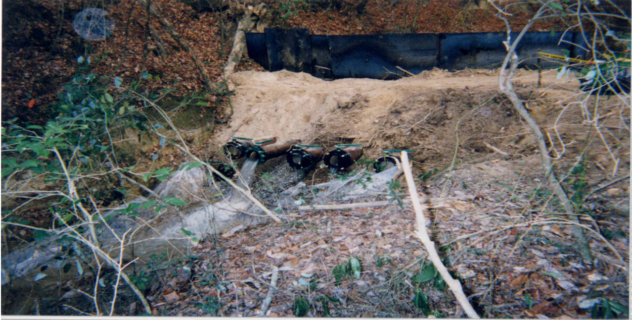
Collins, MS 12/31/99 Site: Area 1A Second Underflow Dam
