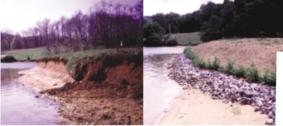
Before-and-after shoreline stabilization efforts at Warrior Path State Park, near Kingsport, Tennessee.
