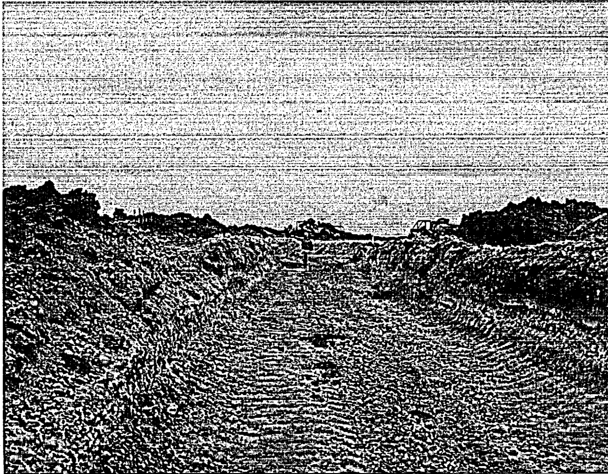
March 10, 1969 – Site Preparation, looking north at first rough grading cut into the turbine area
