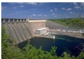
VRAP assesses the vulnerabilities of electric and hydroelectric power generation facilities.
