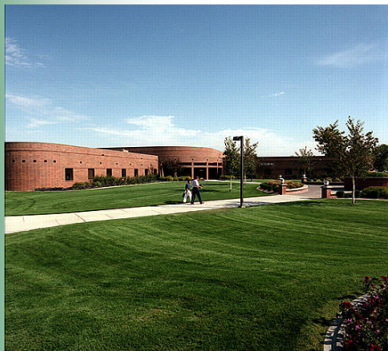
Figure D13.3. Information Sciences Building I
