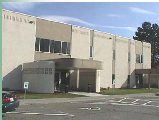
Figure D13.7. 2400 Stevens Building
