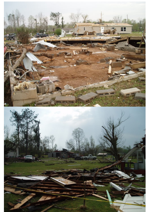
Damage Pictures from the F2 Tornado that struck Yuma, TN
