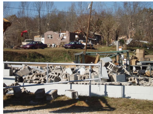
Severe Damage to brick home in Paris, TN
