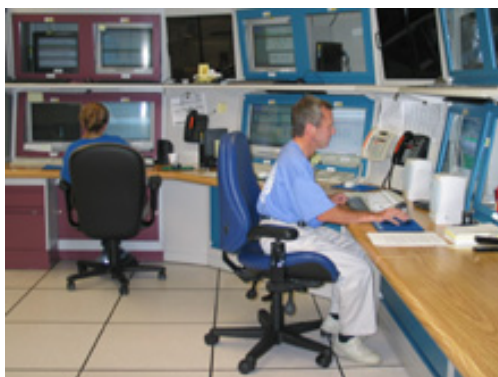
The Control Room at Feynman Computing Center
