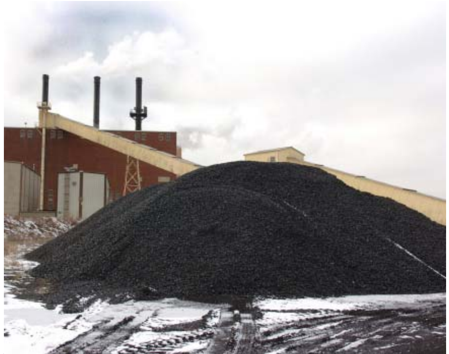
COAL IMPACT – A new report prepared by Argonne’s Environmental Science Division has the potential for far-reaching impacts on the electric utility industry. The report is available online at www.fossil.energy.gov/programs/powersystems/pollutioncontrols/coal_waste_report.pdf .
