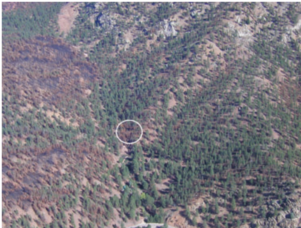
Figure 5 —Aerial view looking north at Lazy Gulch (State Highway 67, northwest of Deckers). The circle indicates where the summer home was destroyed. Note the unburned homes below the circle.
