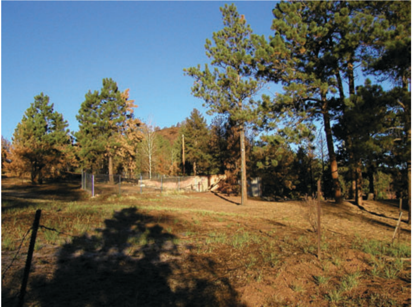
Figure 39 —This home, on the south side of Trout Creek Ranch, was designated as destroyed by surface fire and/or firebrand.
