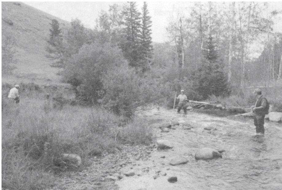
Figure 50. Measuring along the channel centerline and staking.
