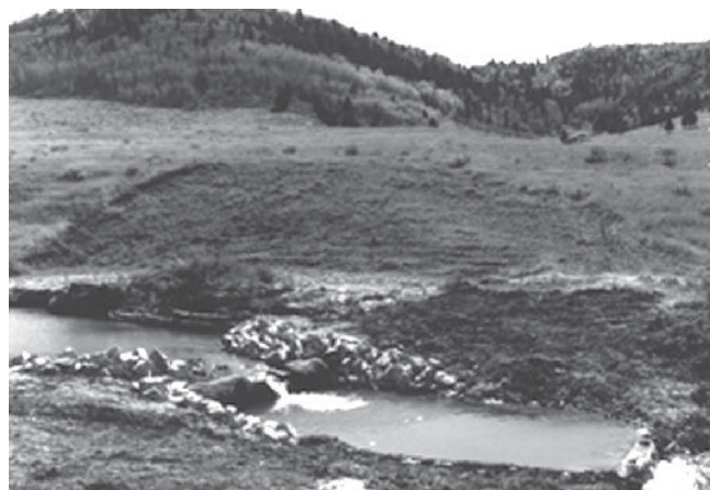
Figure 6 —This disturbed riparian site was broadcast seeded. Shrubs were transplanted along the water's edge. Grazing should be excluded until the disturbance is completely stabilized and the shrubs are fully established and reproducing vegetatively.
