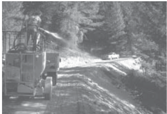
Figure 33 —Hydroseeding roadcuts and fills.
