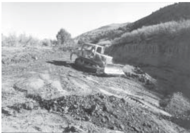
Figure 36 —Three-way dozer reshaping a streambank.
