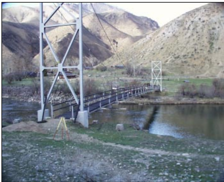
Bernard Bridge repaired after fire damage.
