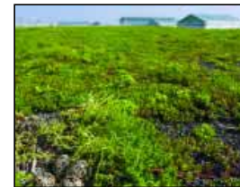
A killdeer ( Charadrius vociferous ) nest of eggs is spotted on the 10.4-ac living green roof at Ford Motor Company's Ford Rouge Center in Dearborn, Michigan. The roof is constructed of a bioengineered stormwater management system that includes drought tolerant sedum and a recycled fabric growing medium. Many innovative solutions have been put into place at the Ford Rouge Center to manage the flow of water on the property in a way that is beneficial to the environment. The use of porous pavement, buffer strips and living green roofs all help to filter and clean stormwater run-off helping protect water quality and providing wildlife habitat.
