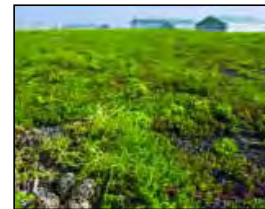
A killdeer ( Charadrius vociferous ) nest of eggs is spotted on the 10.4-ac living green roof at Ford Motor Company's Ford Rouge Center in Dearborn, Michigan. The roof is constructed of a bioengineered storm water management system that includes drought tolerant sedum and a recycled fabric growing medium. Many innovative solutions have been put into place at the Ford Rouge Center to manage the flow of water on the property in a way that is beneficial to the environment. The use of porous pavement, buffer strips and living green roofs all help to filter and clean stormwater run-off helping protect water quality and providing wildlife habitat.
