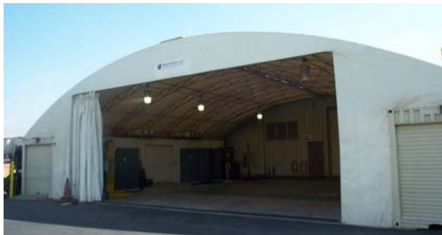
Figure 18. Hydrogen maintenance building
