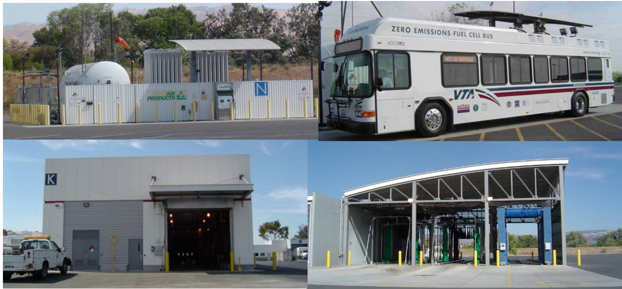
Figure ES-1. Compressed hydrogen dispensing station, fuel cell bus, bus wash, and maintenance facility
