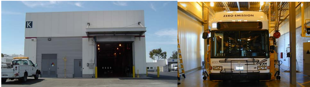
Figure 11. Maintenance facility used for the fuel cell buses at VTA
