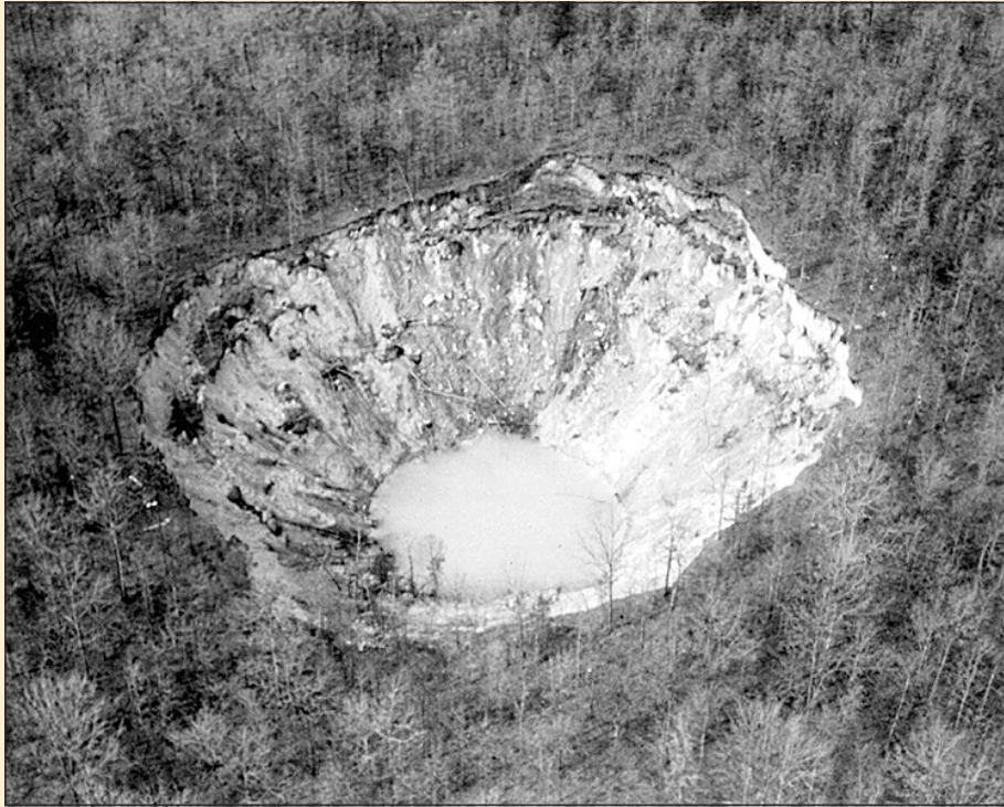
Figure 23. The “December giant,” a large sinkhole, developed rapidly in Shelby County, Alabama, in December 1972. The sinkhole measures 145 m long, 115 m wide, and 50 m deep. (USGS Photographic Library-USGS #140.)
