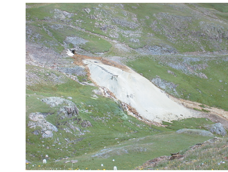
Figure p7. Roy Pray mine adit and dump. Note rails (gray linear feature on upper left side of dump) for scale. Width of dump is about 50 meters.
